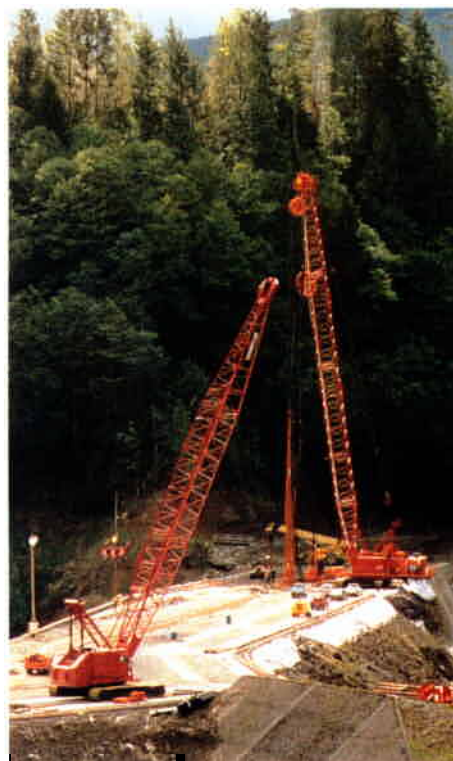
DAM VIEWED FROM RIGHT BANK
