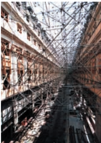
Struts to outer walls
