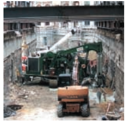
HL 4000 Compact Hydrofraise building diaphragm wall
