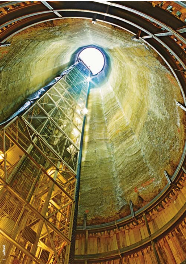
< 65 m of shaft seen from the bottom of the shaft. The rib and timber supports can be seen at the foot of the D. Wall
