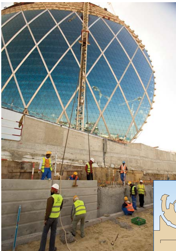
Precast fascia panels installation
