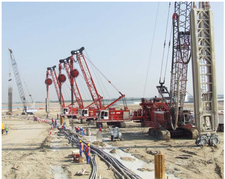
KS and hydrofraise along the future quay wall of Khor Al Raha
