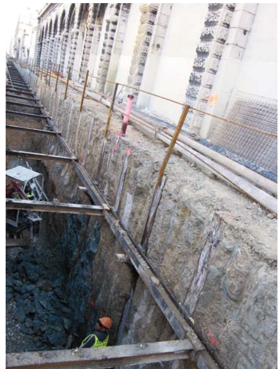
The Geomix wall > during earth moving work
