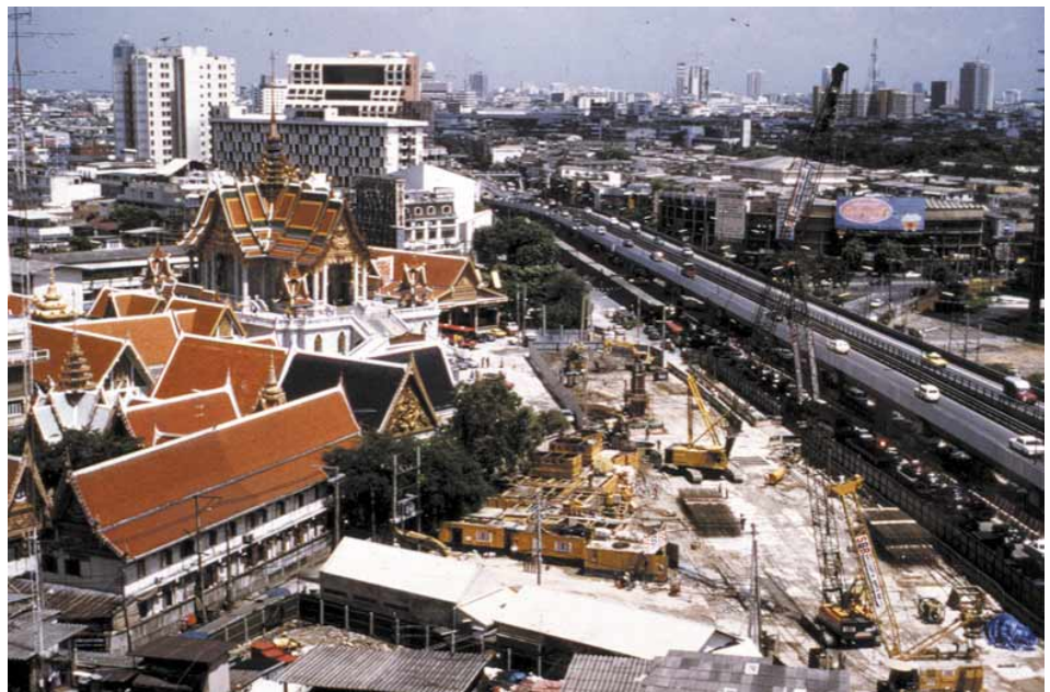
View of work at Samyan station
