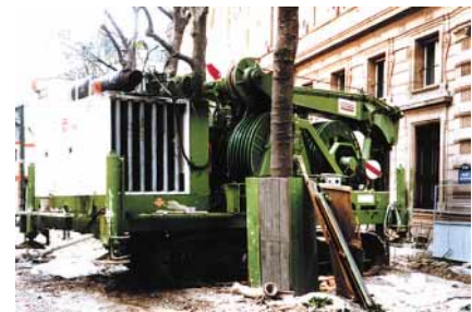
Latine Hydrofraise at work
