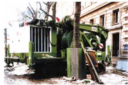
Latine Hydrofraise at work
