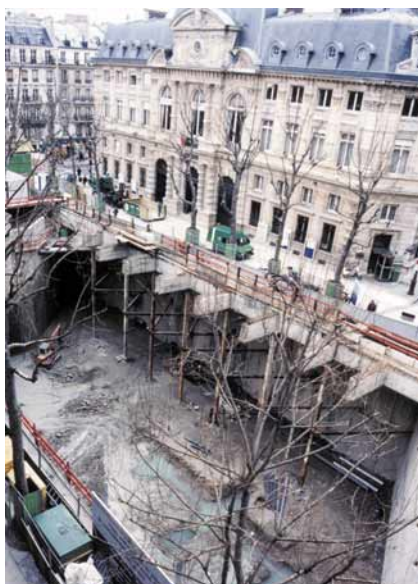
Place Baudoyer during and after construction
