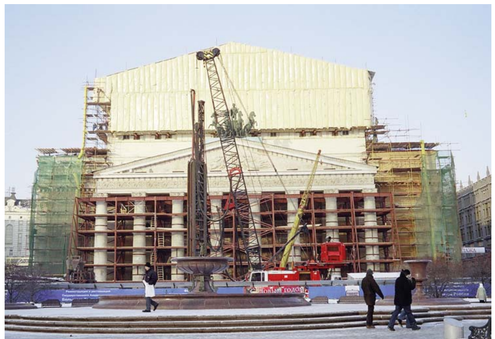
Hydrofraise in front of the facade of the Bolchoi
