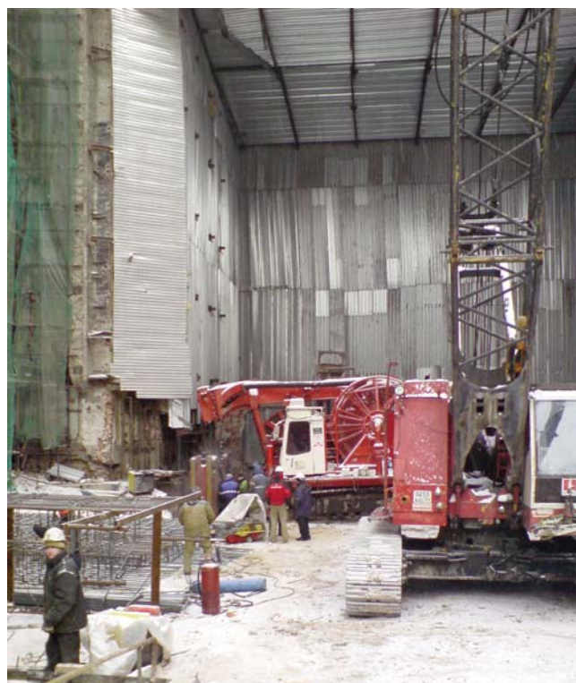
Hydrofraise “latin” working inside of “Bolchoi”
