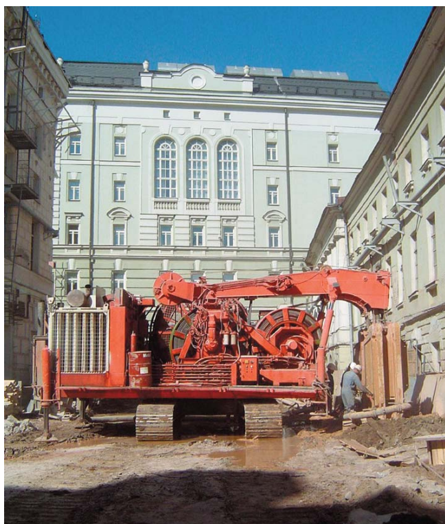
The Hydrofraise “Latine” was used due to its compact design
