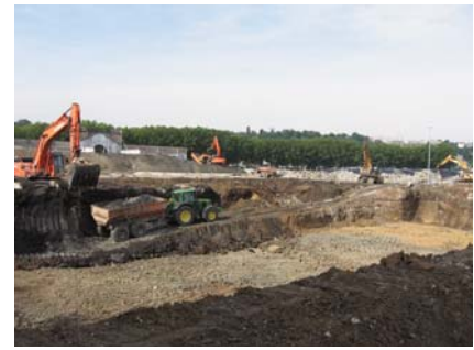
Extraction of materials above the water table
