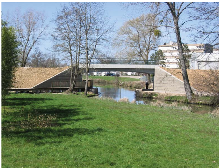
New Reyssouze bridge
