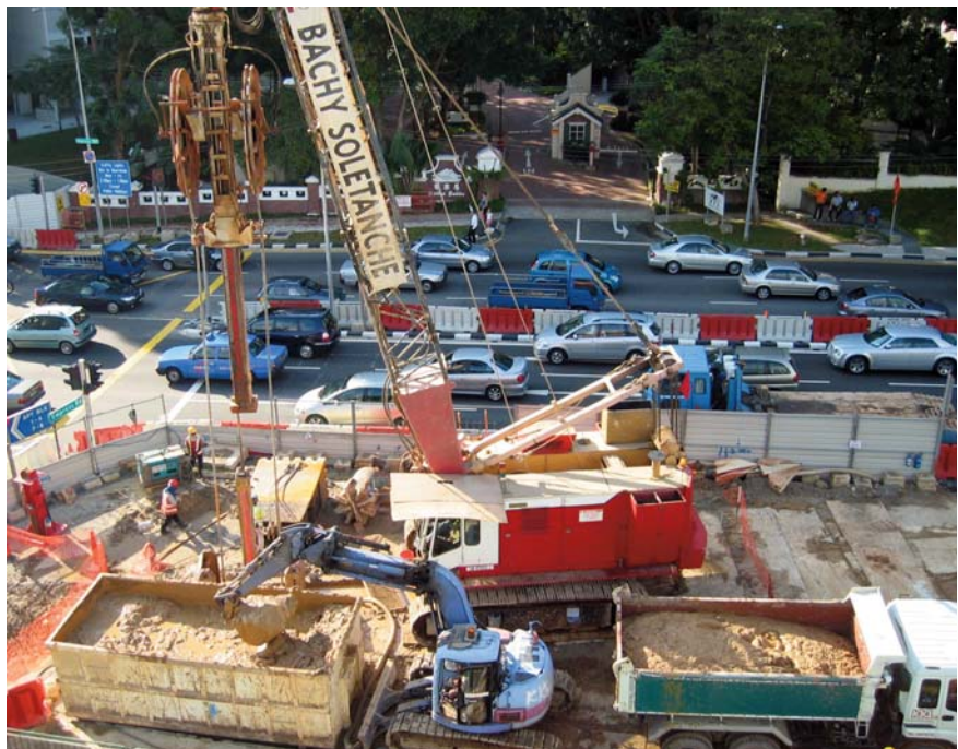
KS3000 Hydraulic Rig working parallel to the diaphragm wall
