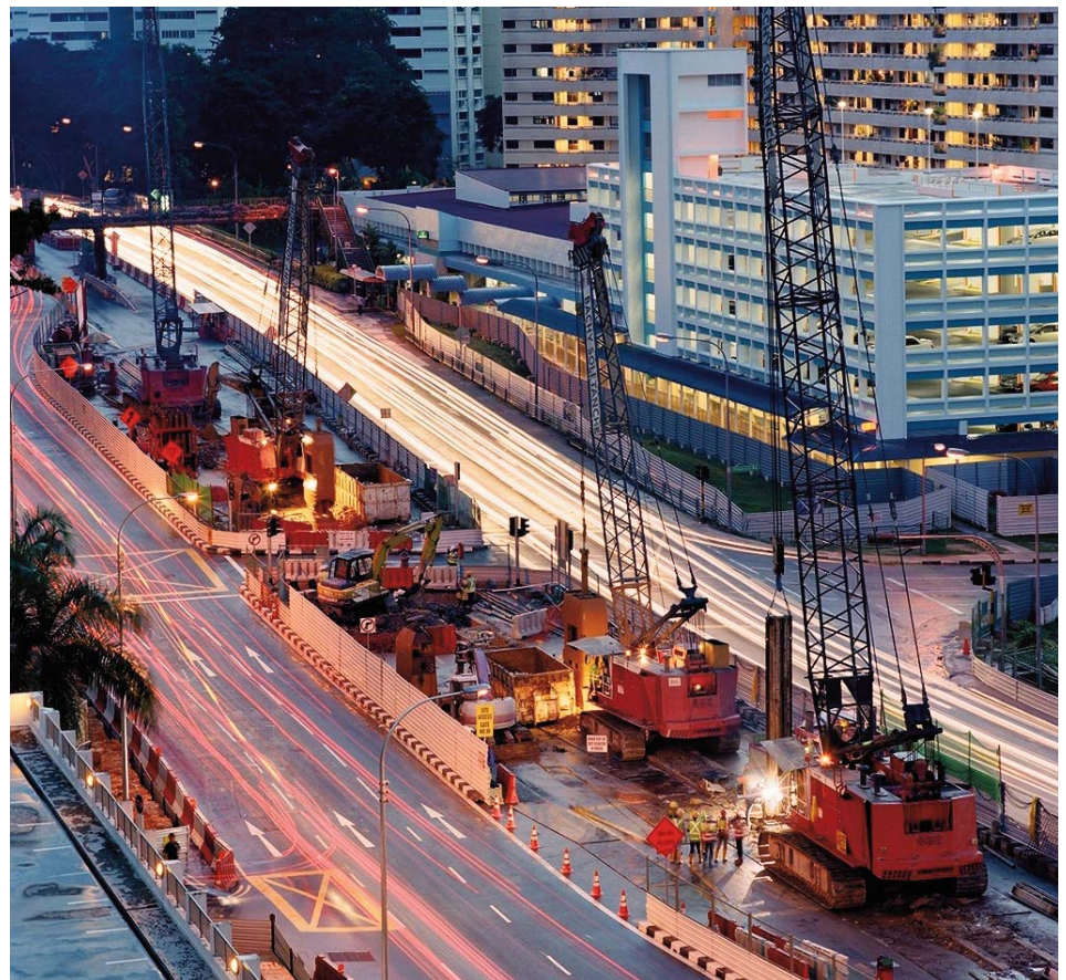
Excavation of the diaphragm wall within a 'traffic island'
