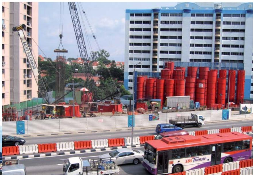
*General view of the bentonite plant and the construction of the retaining walls for a station entrance*
