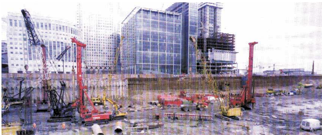
Construction work in progress
