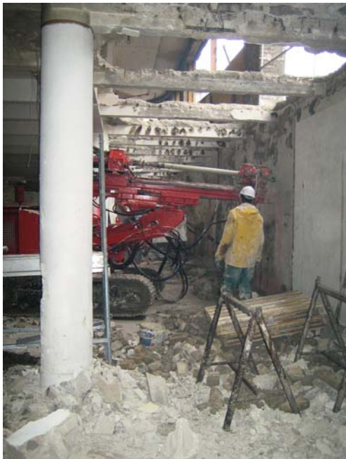
< Installing the ground anchors in the existing basement
