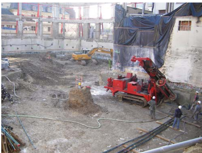
The ground anchors were installed as the earthworks progressed
