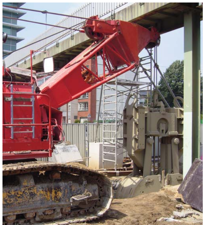
Constructing the wall under limited headroom
