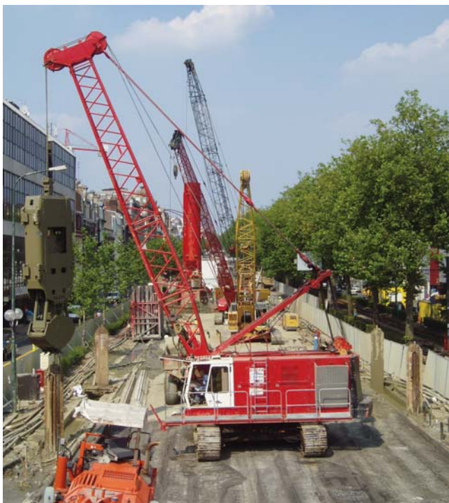
Constructing the diaphragm wall
