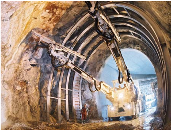
MONACO T33 tunnel
