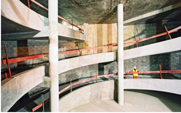
FRANCE - Boulogne-Billancourt Seguin car park
