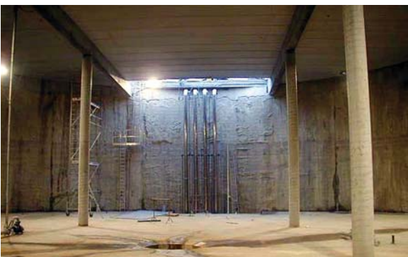
FRANCE - Anglet Pechmeja storm tank
