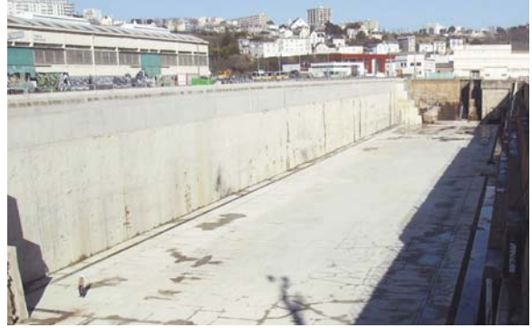
FRANCE - Brest Dry dock n°1
