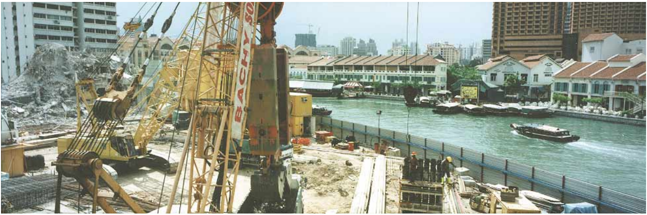
General view of diaphragm wall excavation adjacent to the Singapore River
