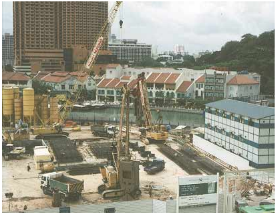
KS and cable grab operations underway
