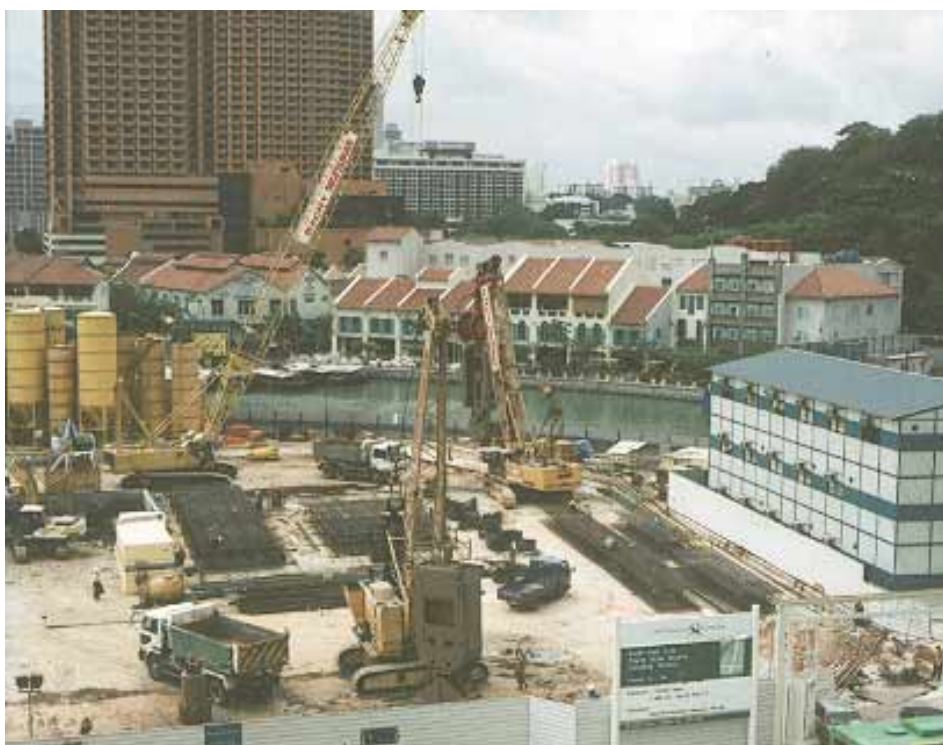
KS and cable grab operations underway
