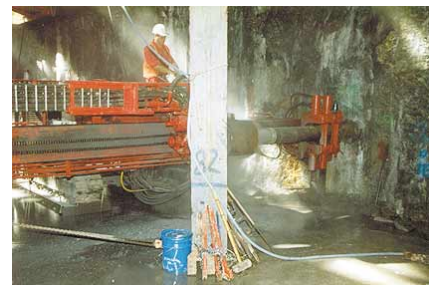
Jet grouting under progress
