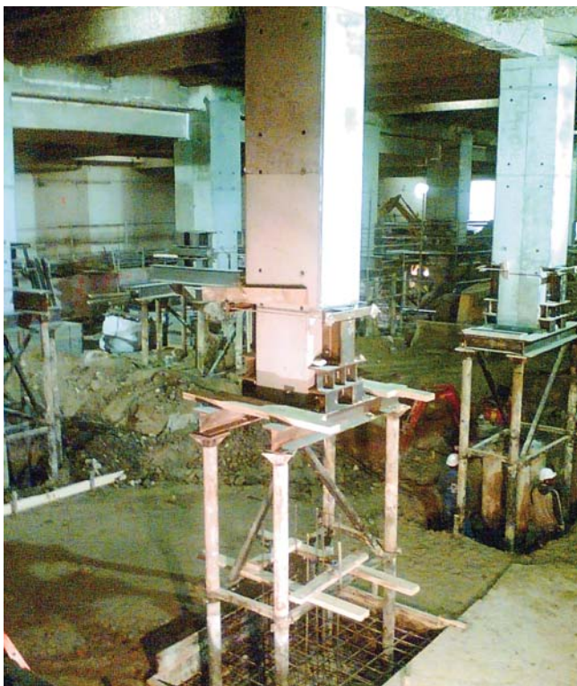
Column underpinning micropiles
