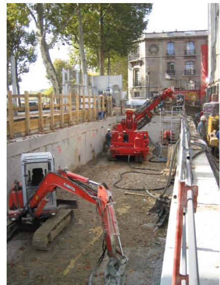
Earth moving and Ground anchors
