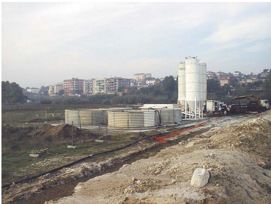
View of site during construction
