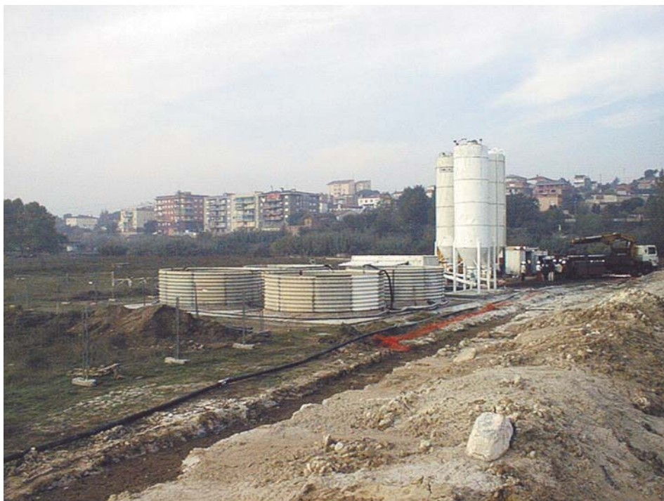
View of site during construction
