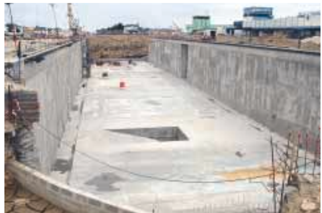
Dock after pouring reinforced concrete floor
