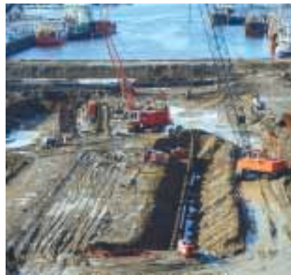
Diaphragm wall and sheet pile driving
