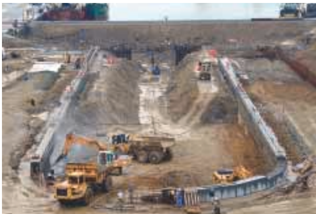
Capping beam and sidewalls
