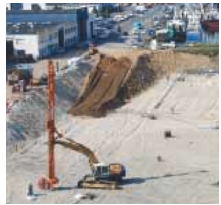
Sinking strip drains
