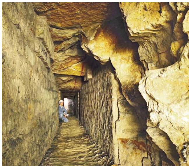
View of a brick lined tunnel
