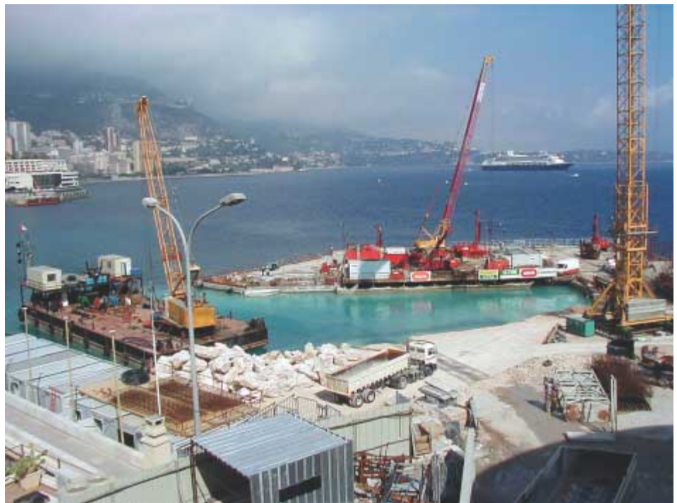
View of jobsite
