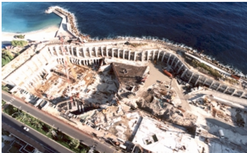
Overall view of the site (diaphragm wall with buttresses, T walls, slabs)
