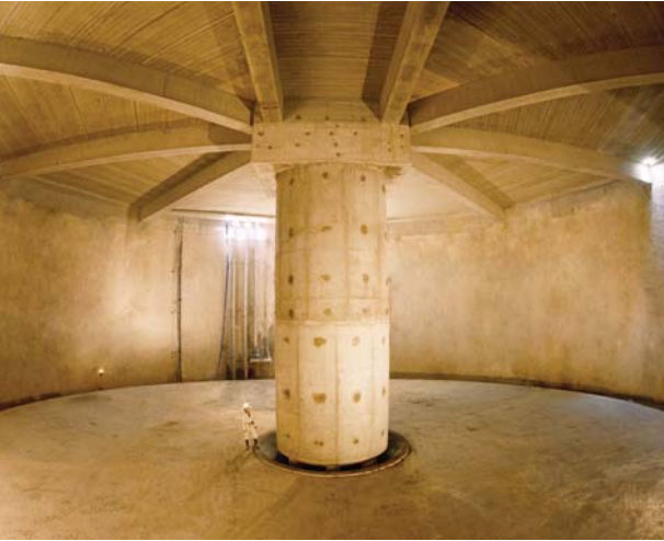
Self-stabilising circular wall for an underground reservoir.
