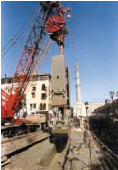
Diaphragm wall being built at El Hussein station
