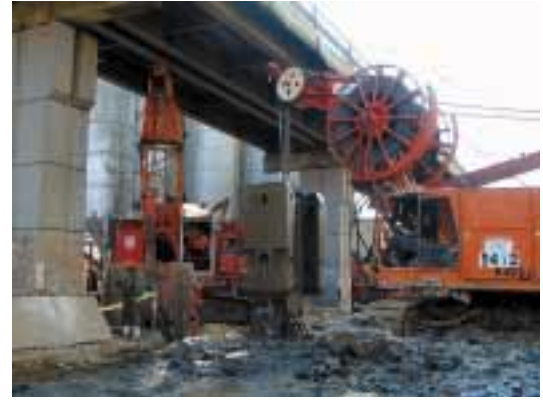
Diaphragm wall for Attaba TBM arrival shaft being built under fly-over
