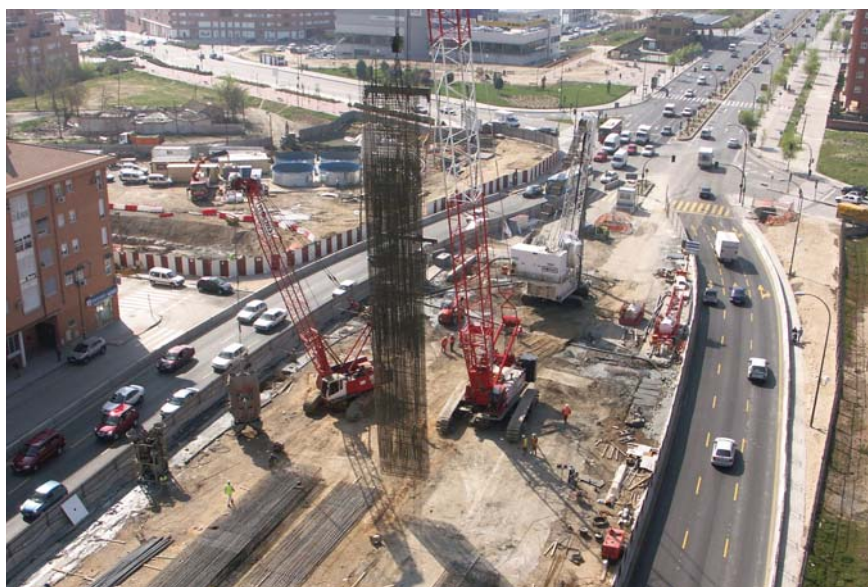
Steel reinforcement
