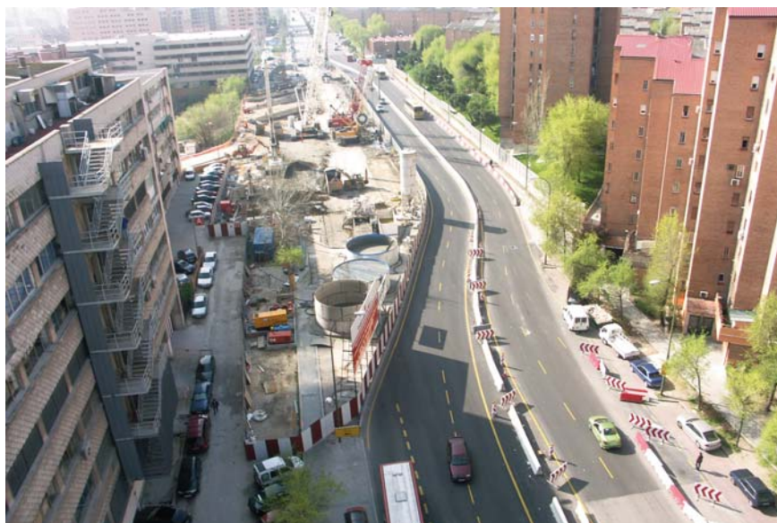
General view of the site
