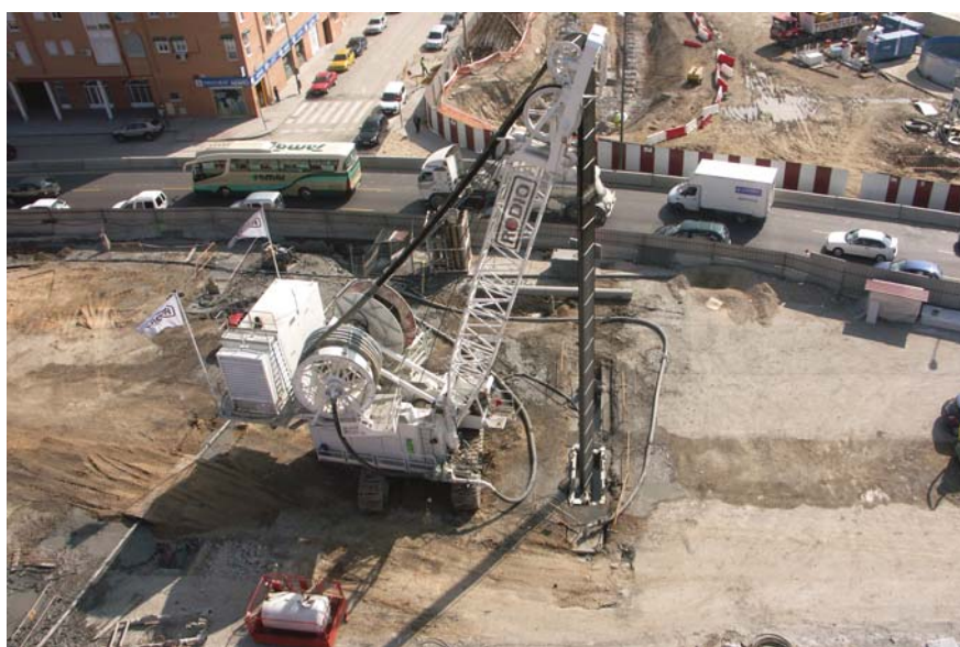
Hydrofraise excavating a D.W. panel
