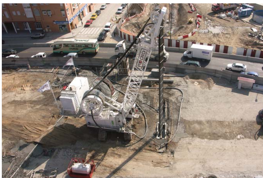
Hydrofraise excavating a D.W. panel
