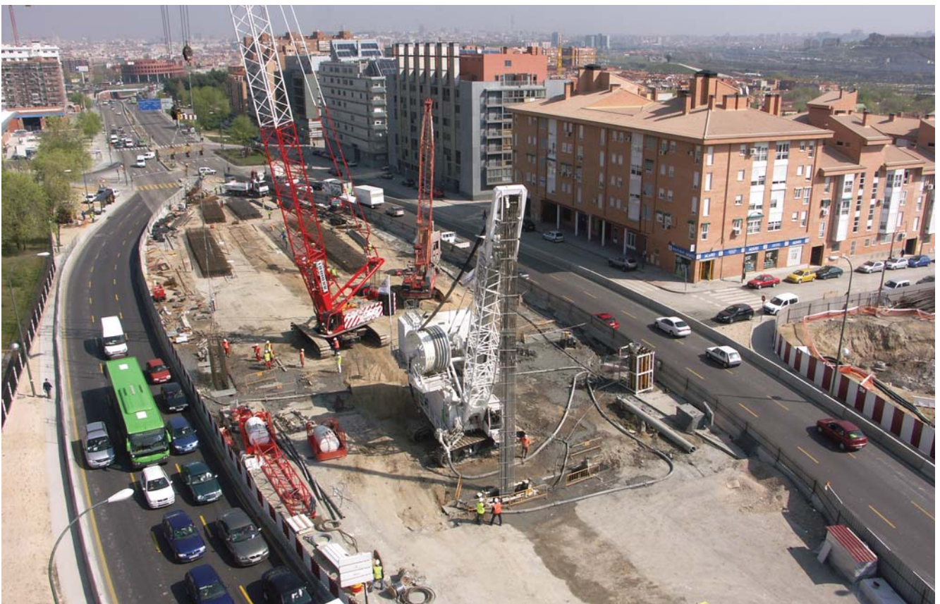
General view of the site
