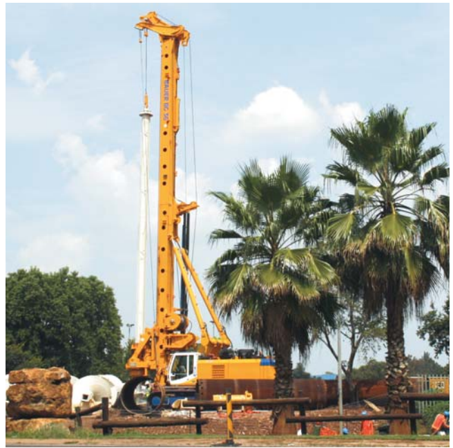
BG 36 drilling rig
