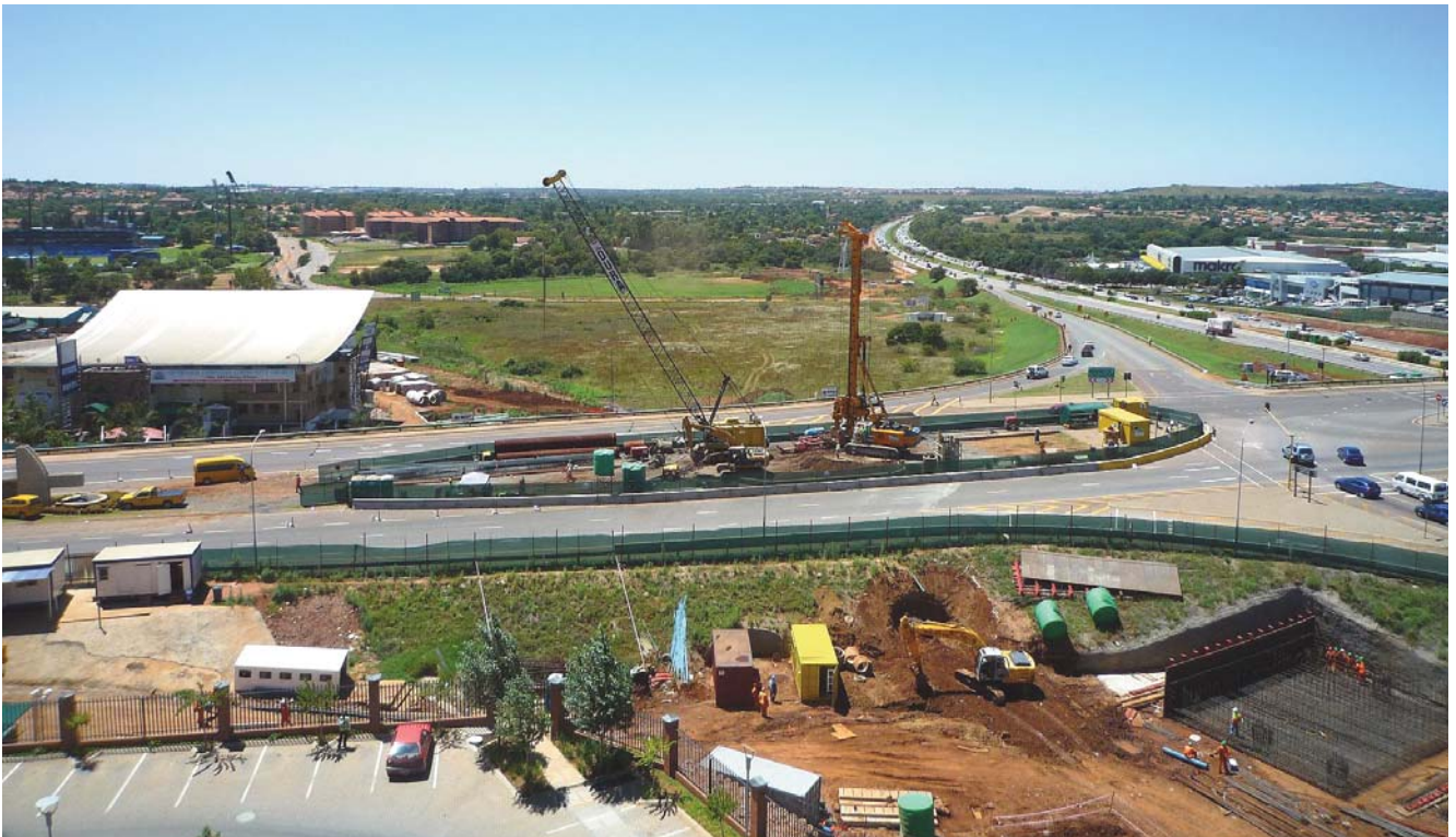
Constructing piles on pier no 12b
