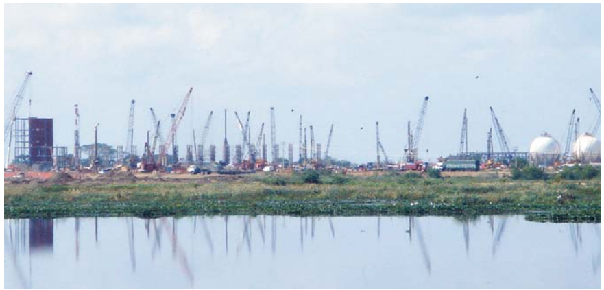
Site overview with its forest of cranes
