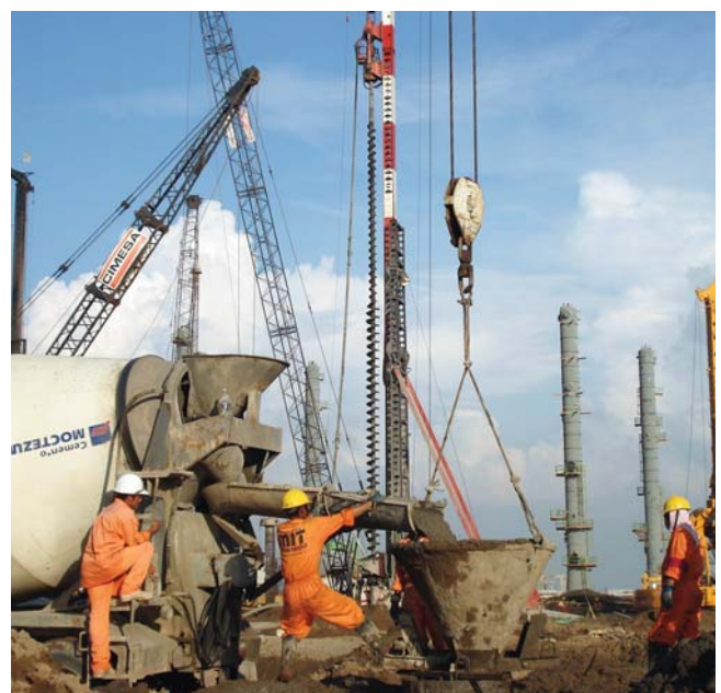
Pile concreting
