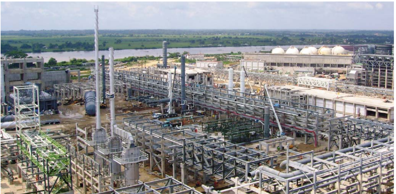
View of the refinery during construction
