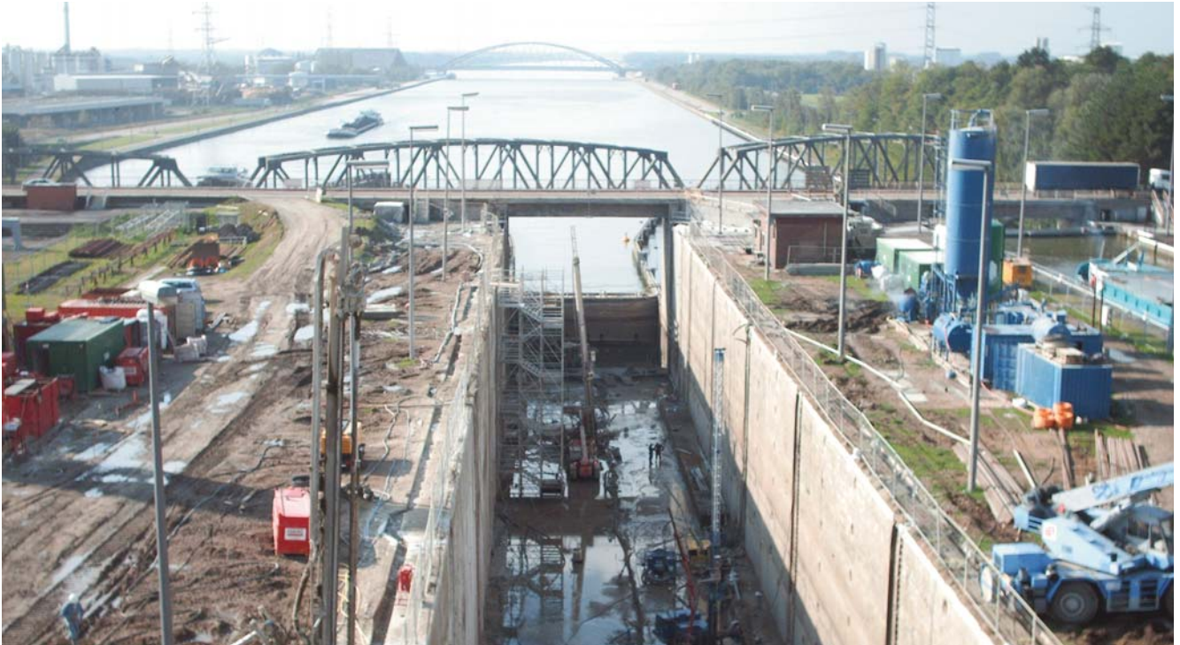
Central lock: stabilization work
