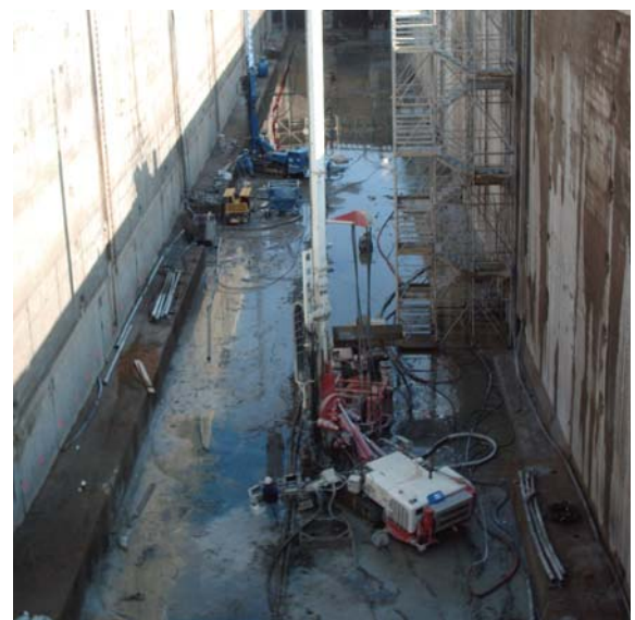
Jet grouting under the slab
