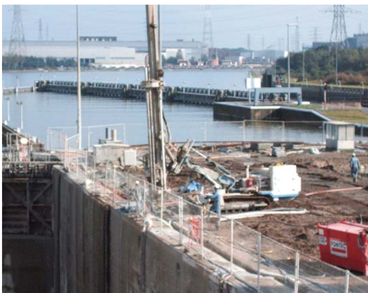
Anchors in the side walls
