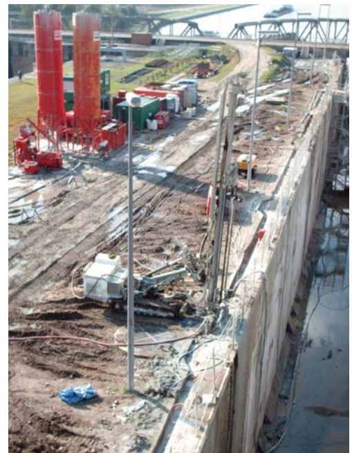
Jet grouting plant and drilling operation
