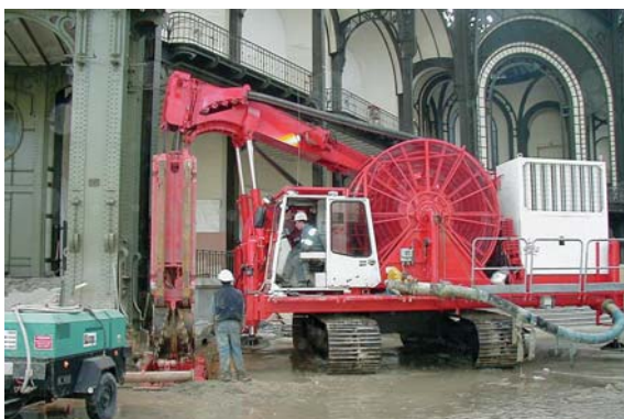
Installing the diaphragm wall
