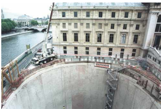
Completed circular diaphragm wall
