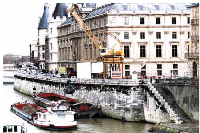
Spoil disposed of directly by barge
