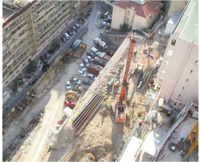
Construction of working piles in the Plati zone
