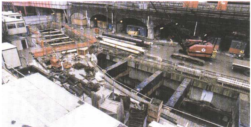
Waterloo Link during construction
