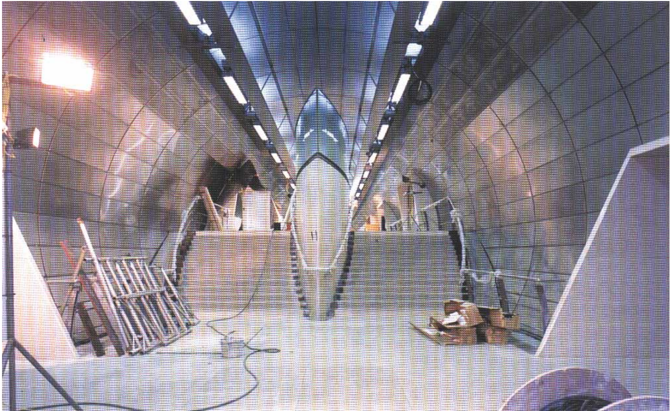
Completion work being carried out on station tunnel concourse
