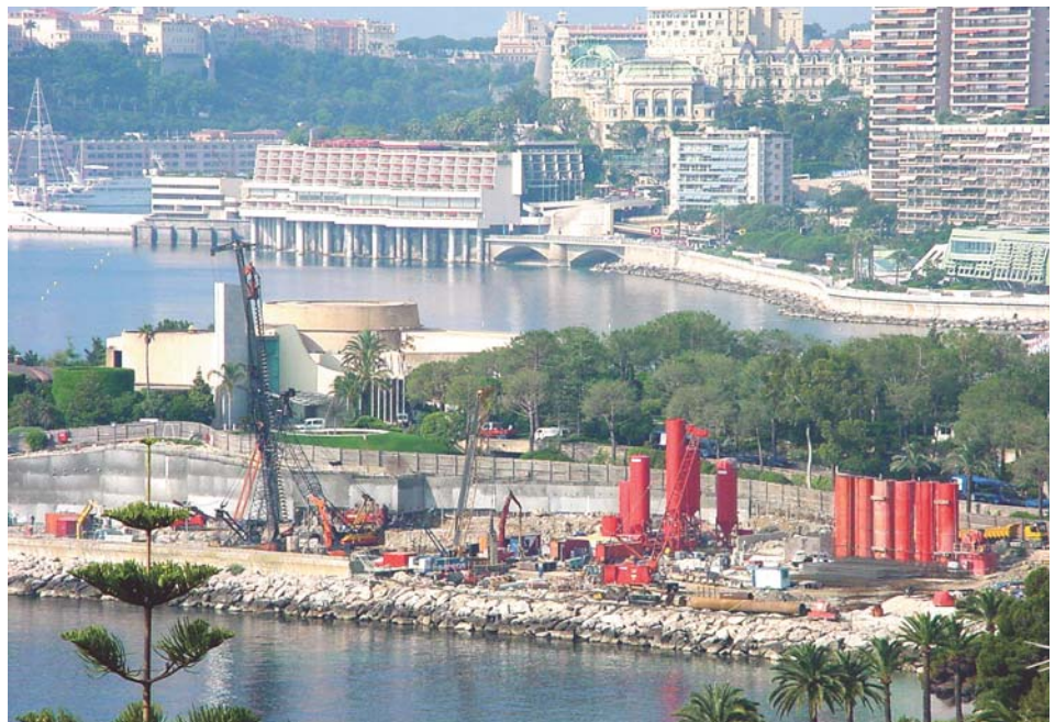
General view of the worksite
