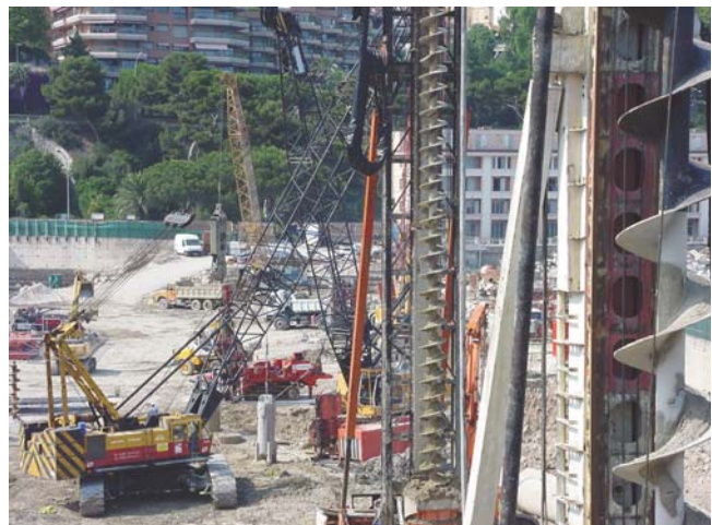
Foundation pile works
