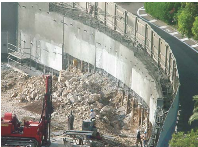
Diaphragm wall works
