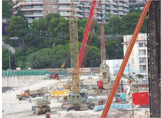
Foundation support pile works
