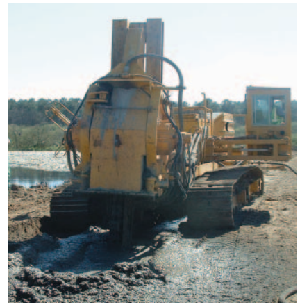
Barrier using soil mixing built with the Trenchmix® trencher
