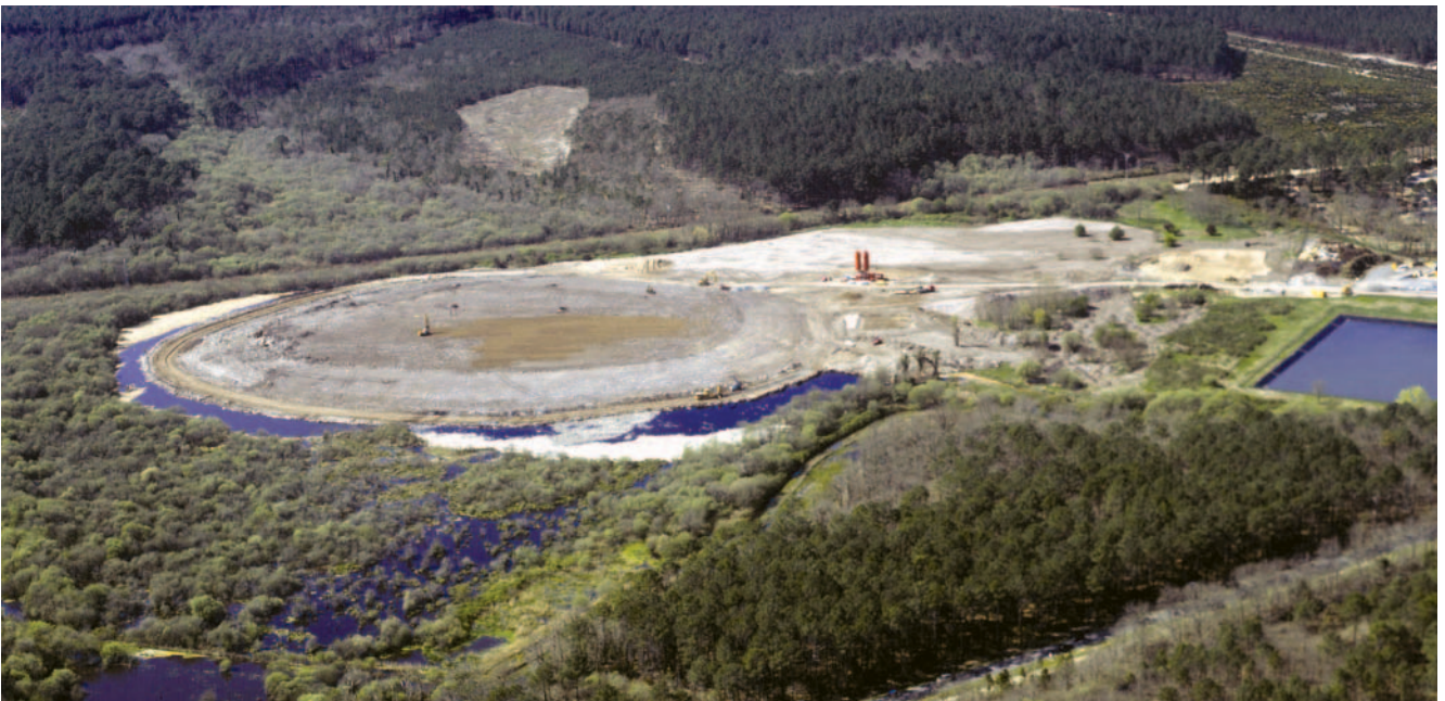
Overall view of construction site
