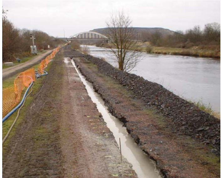
View of the site
