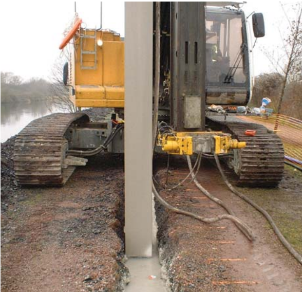
Construction of a thin cut-off wall by vibwall technique
