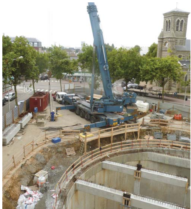
Overview of works in progress
