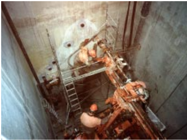
Drilling horizontal boreholes
