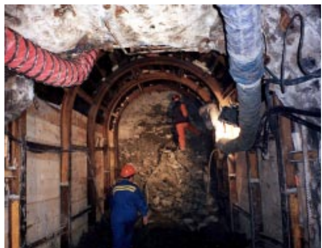
Access tunnel in progress
