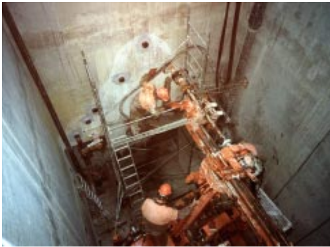
Drilling horizontal boreholes
