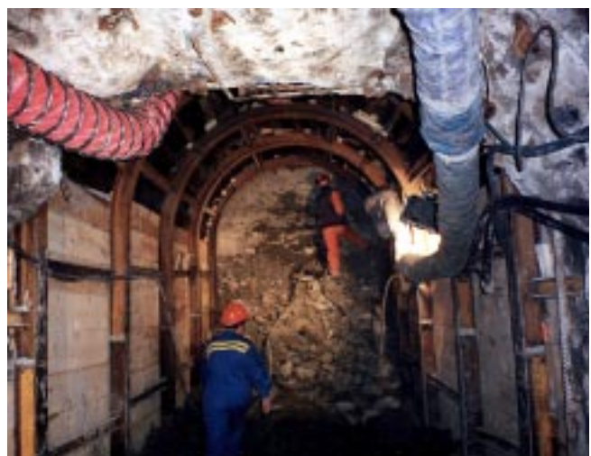
Access tunnel in progress
