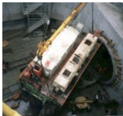
Lowering of TBM element
