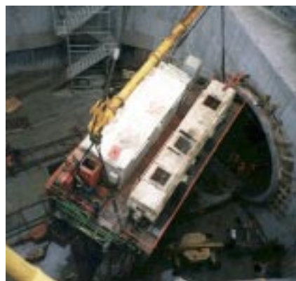
Lowering of TBM element
