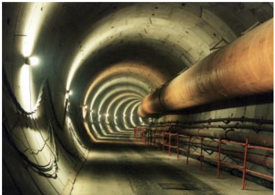
Tunnel section with roadway poured behind face
