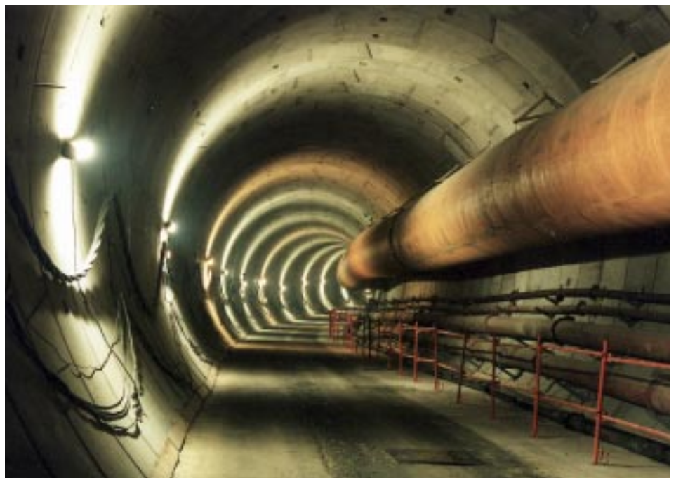
Tunnel section with roadway poured behind face
