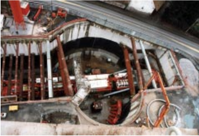
Erecting TBM at Louis Constant station
