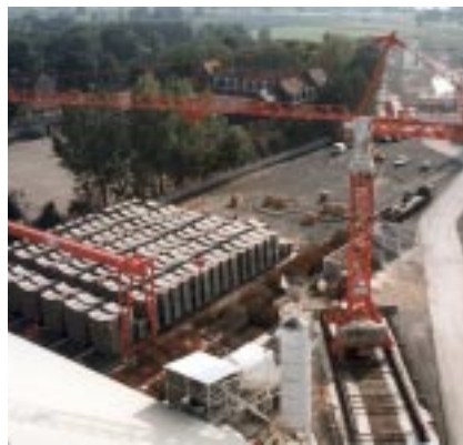
Lining segment casting and storage
