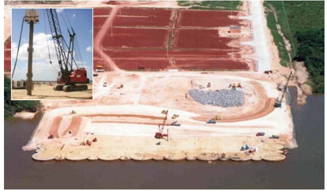
Vibrocompaction of the backfill
