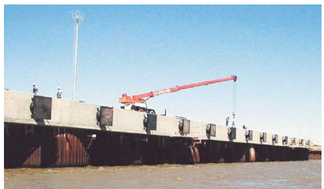
Front view of the quay and its defence structures
