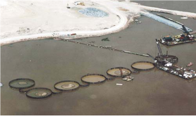
Construction of caisson n°8 and of the west cofferdam
