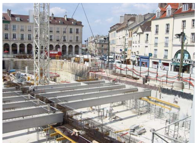
Beam installation to construct the cover slab
