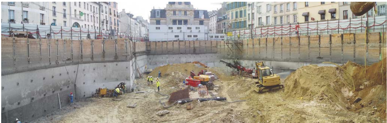
Earthworks and construction of the concrete sprayed wall with stabilising nails
