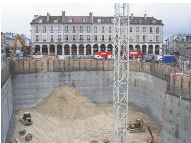
View of the floor of the excavation on the Arcades side
