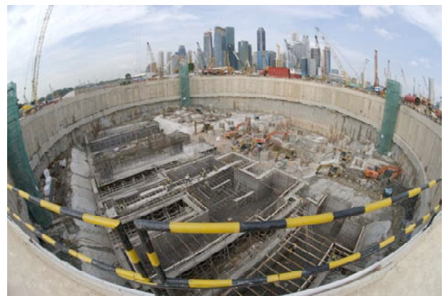
Pile caps under construction within the Tower One 'doughnut'
