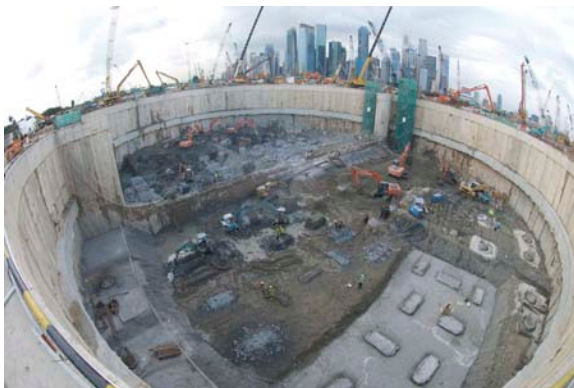
Bulk excavation of the 'peanut'
