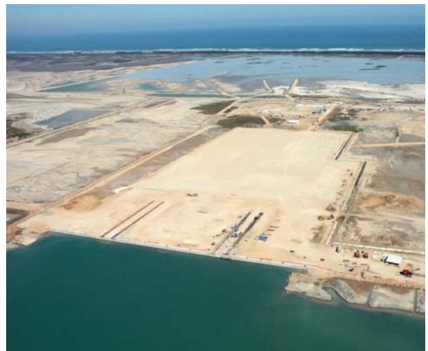
MEXICO - Altamira Oil platform construction terminal
