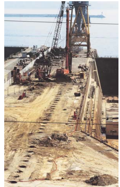
FRANCE - Dunkerque Charles de Gaulle Lock Underpinning
