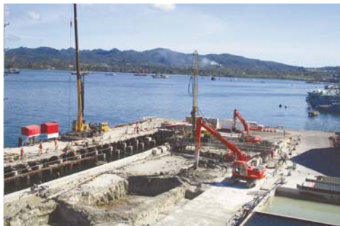
FIJI - Fiji Island Quay wall refurbishment
