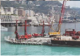
MONACO - La Condamine Port Soil improvement under caisson
