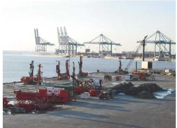
BELGIUM - Anvers Quay underpinning
