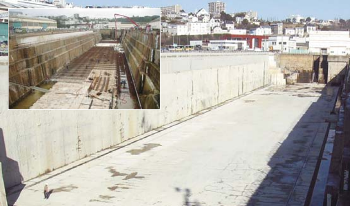
FRANCE - Brest - Dry dock n°1 Widening and modernisation
