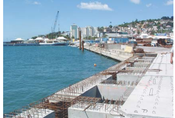
FRANCE - Fort de France - Pointe Simon Terminal
