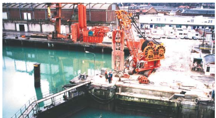
FRANCE - Dieppe Lock widening and deepening
