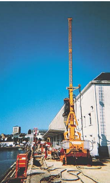
FRANCE - Concarneau Quay underpinning
