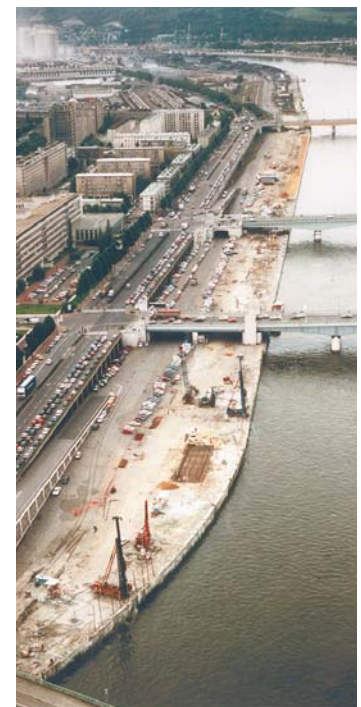
FRANCE - Rouen Refurbishment of the quays
