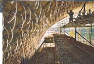
← FRANCE - Paris - Pont Royal Reinforcement of the arches
