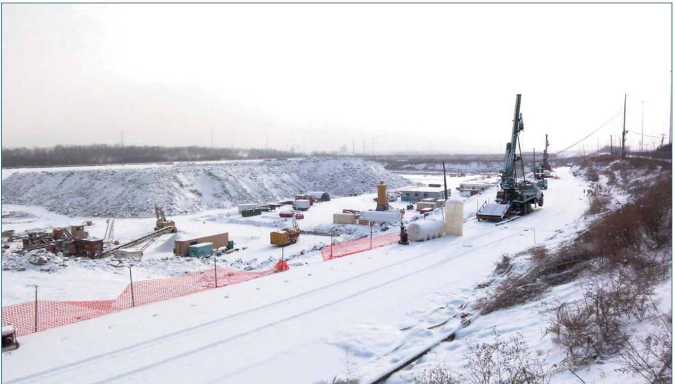
Sonic core drilling machines on the working platform
