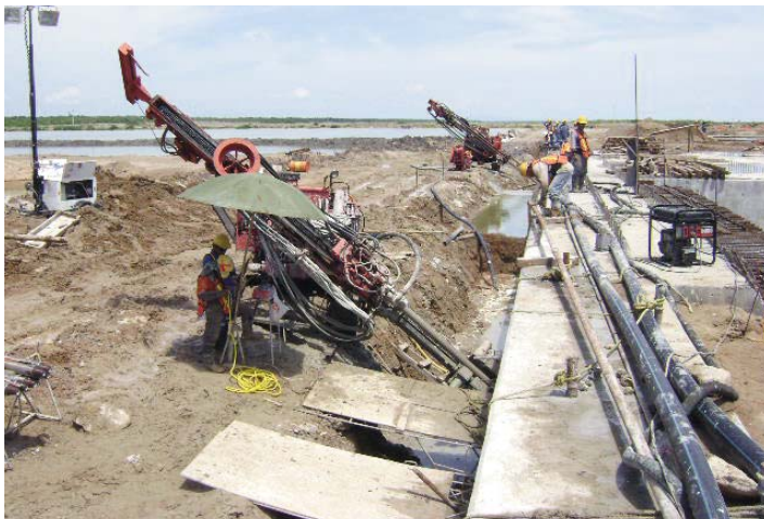
Drilling and fitting the ground anchors
