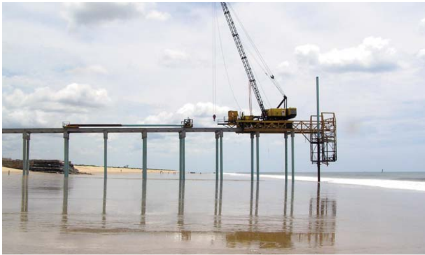
Pile transport in progress
