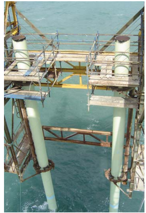
Driving guide for a couple of piles
