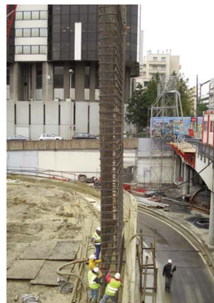
Installation of the reinforcement cages
