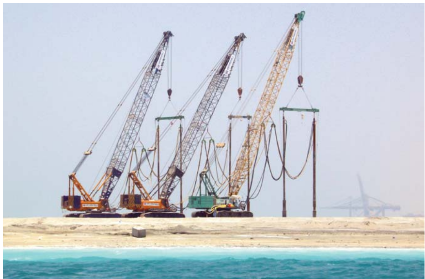
Vibrocompaction tandem unit in action. 15m depth of treatment
