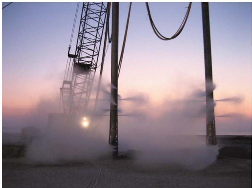
Vibrocompaction tandem unit in action. 15m depth of treatment
