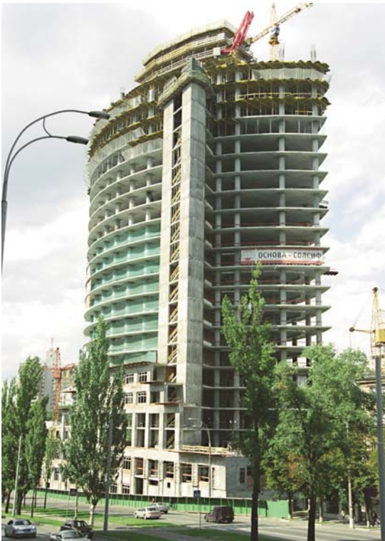
Construction of the 131 meter high tower
