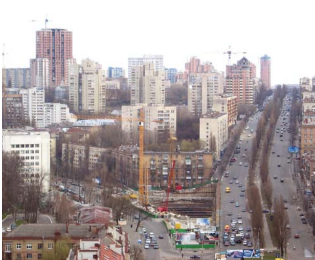
The excavation between Lesi Ukrainky boulevard and Mechnykova street
