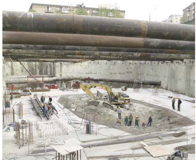
The ring slab under the struts
