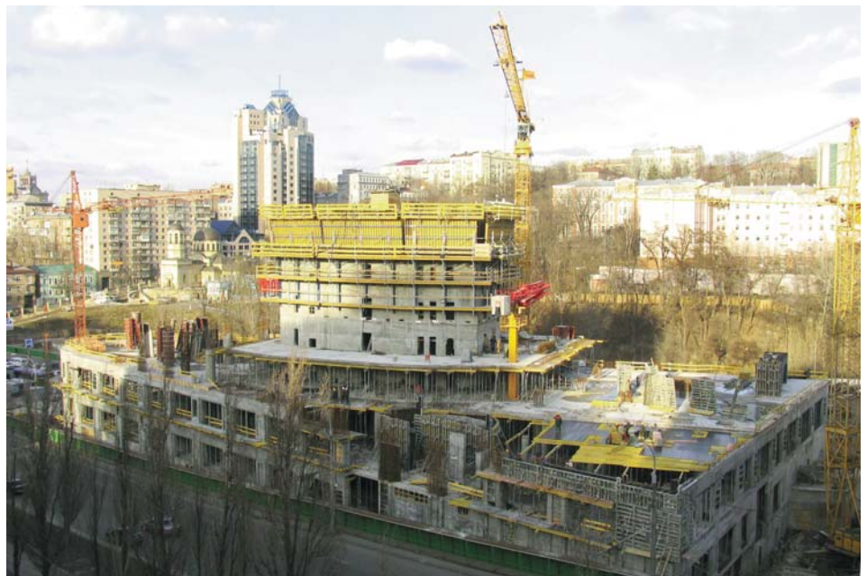
Start of the superstructure
