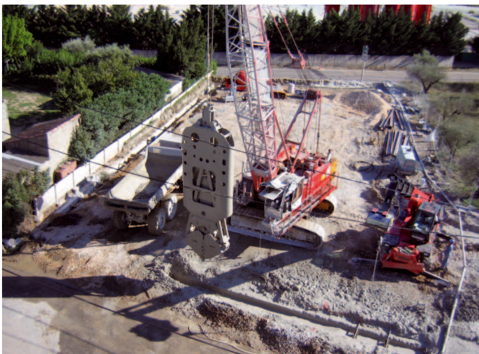
General view of the wall construction site
