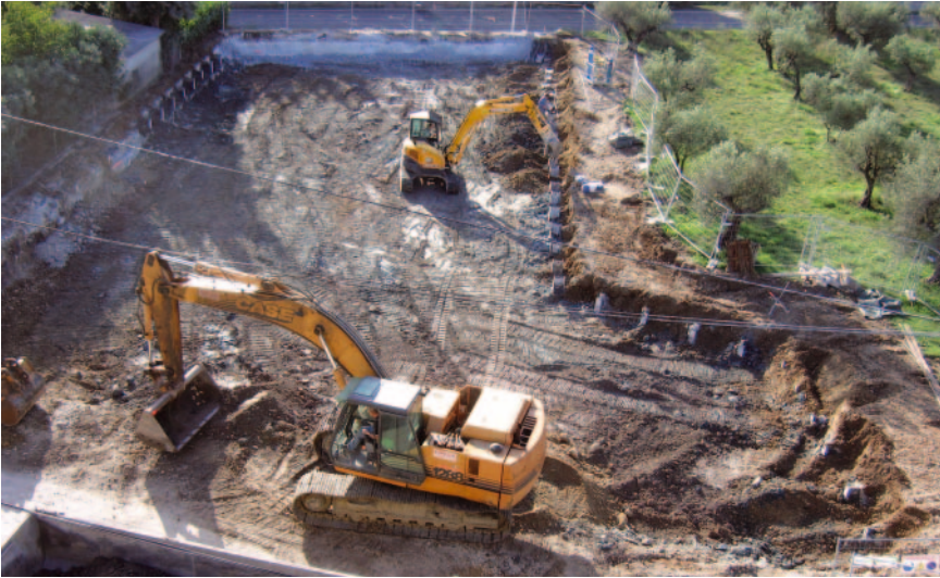
Earthworks up to the level of the waterproofing system
