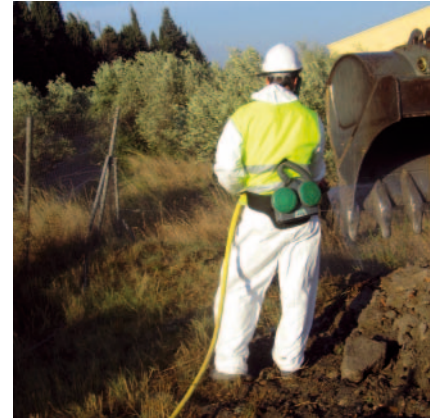
Watering of the earth during the earthworks
