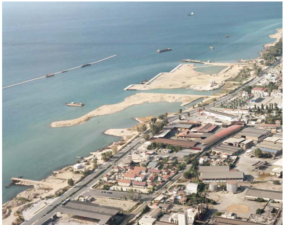
General view of site
