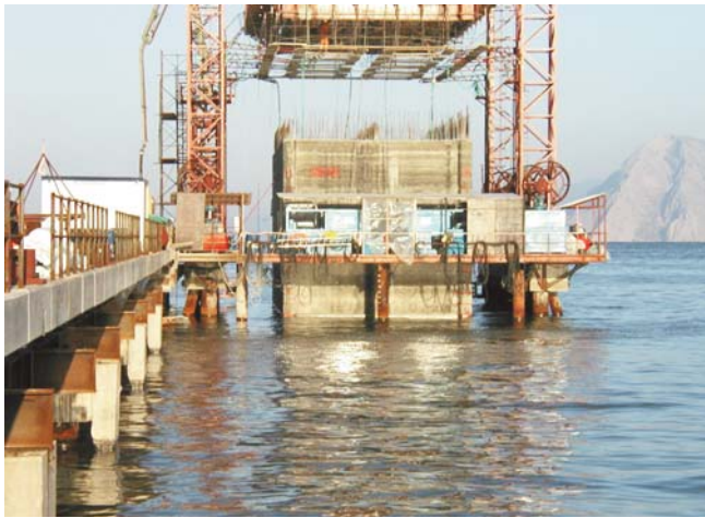
Caisson construction
